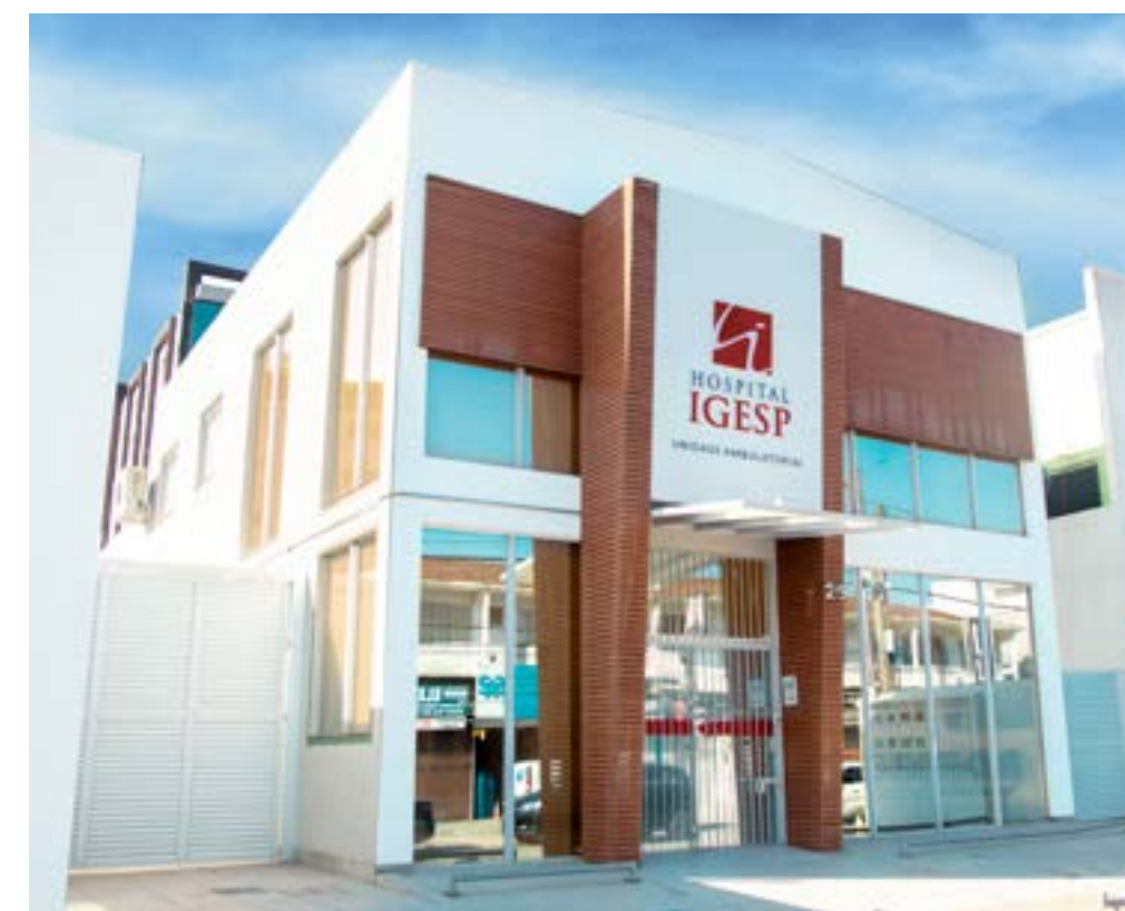
IGESP Guarujá Rua Montenegro, 25
